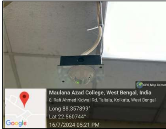
MOTION SENSORS FOR LIGHTS INSTALLED AT SEMINAL HALL AND LOBBY OF PRINCIPAL'S ROOM
