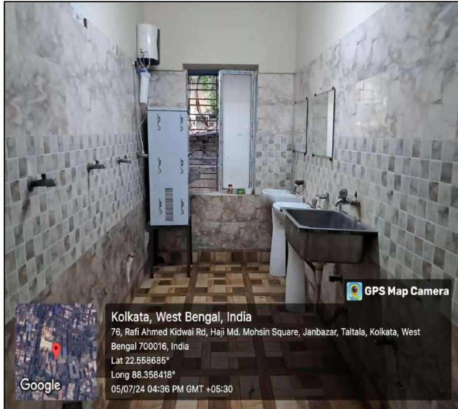
WELL MAINTAINED WASH BASINS
