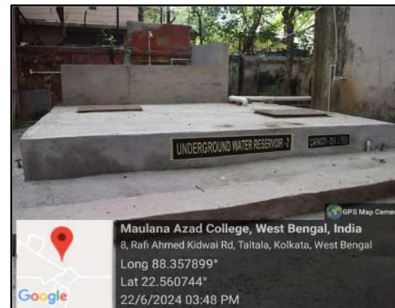
UNDERGROUND WATER RESERVOIR 2 (33K LTS. CAPACITY)
