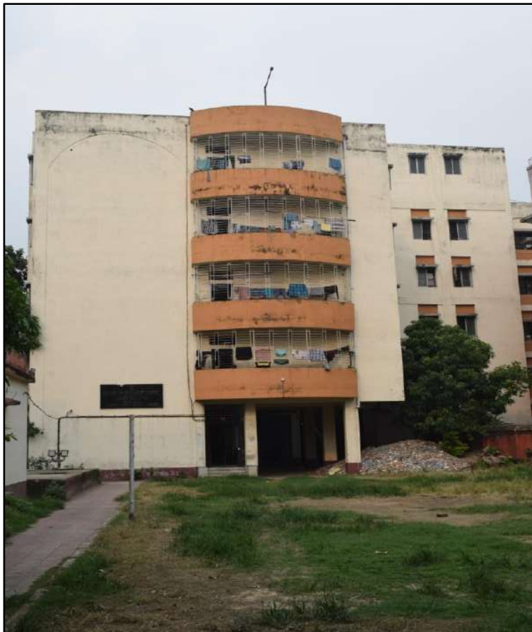
ANNEX BUILDING OF BOYS' HOSTEL
