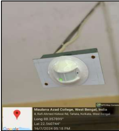
MOTION SENSORS FOR LIGHTS INSTALLED AT SEMINAL HALL AND LOBBY OF PRINCIPAL'S ROOM
