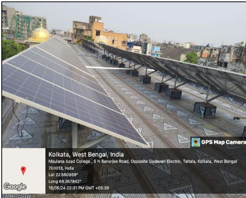
INSTALLED SOLAR PANEL ON COLLEGE ROOFTOP
