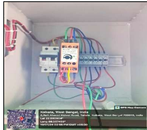
SENSOR BASED AUTO CUT PUMP MOTOR SET IN WATER TANK
