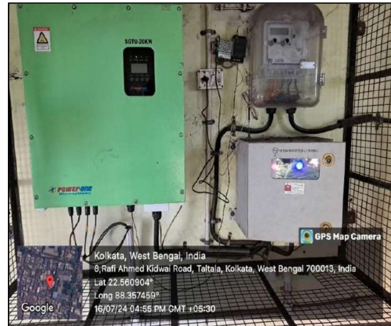
WHEELING TO THE GRID
