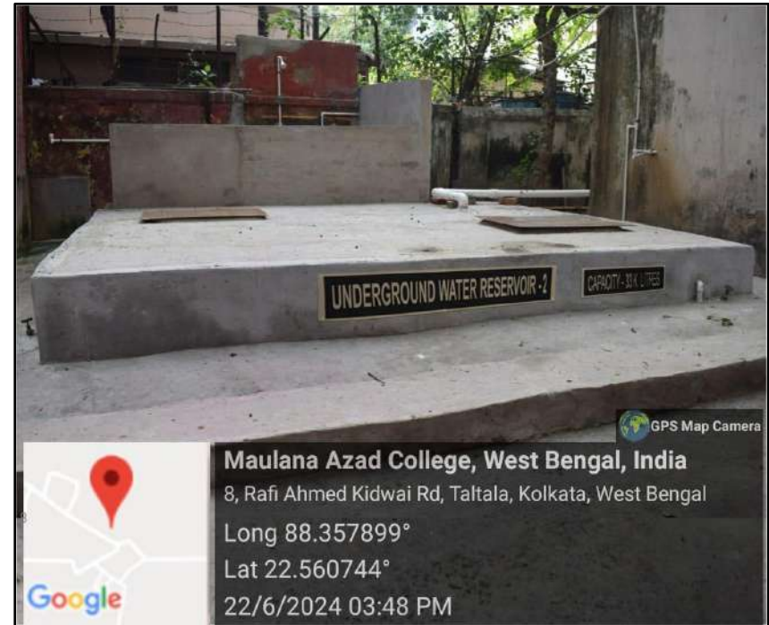
UNDERGROUND WATER RESERVOIR 2 (33K LTS. CAPACITY)
